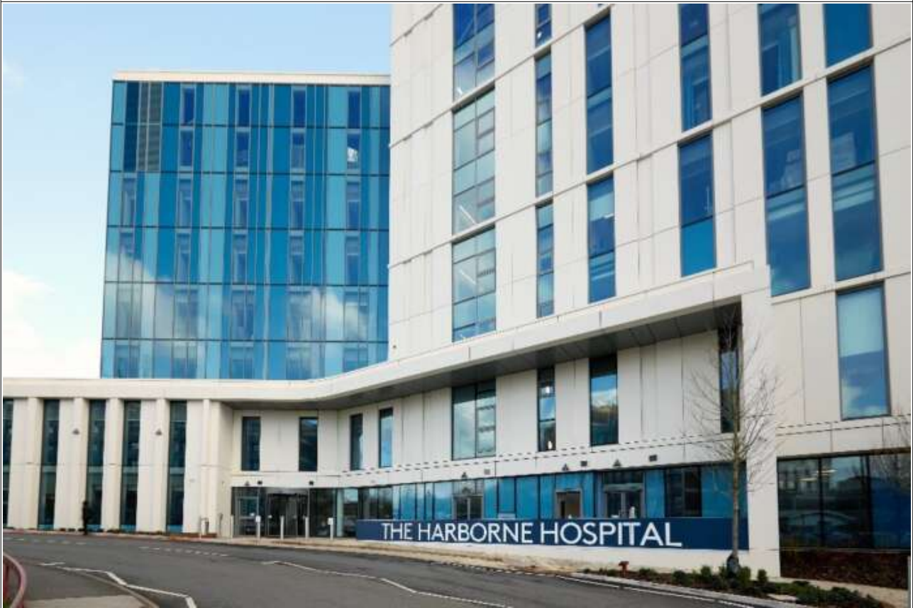
The Harborne Hospital Birmingham Mindelsohn Way, Birmingham, B15 2TQ
